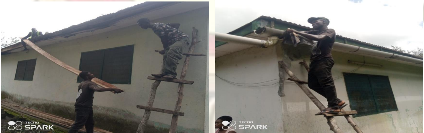
Figure 7.5: Repair of Rain gutters at Zitoe camp
